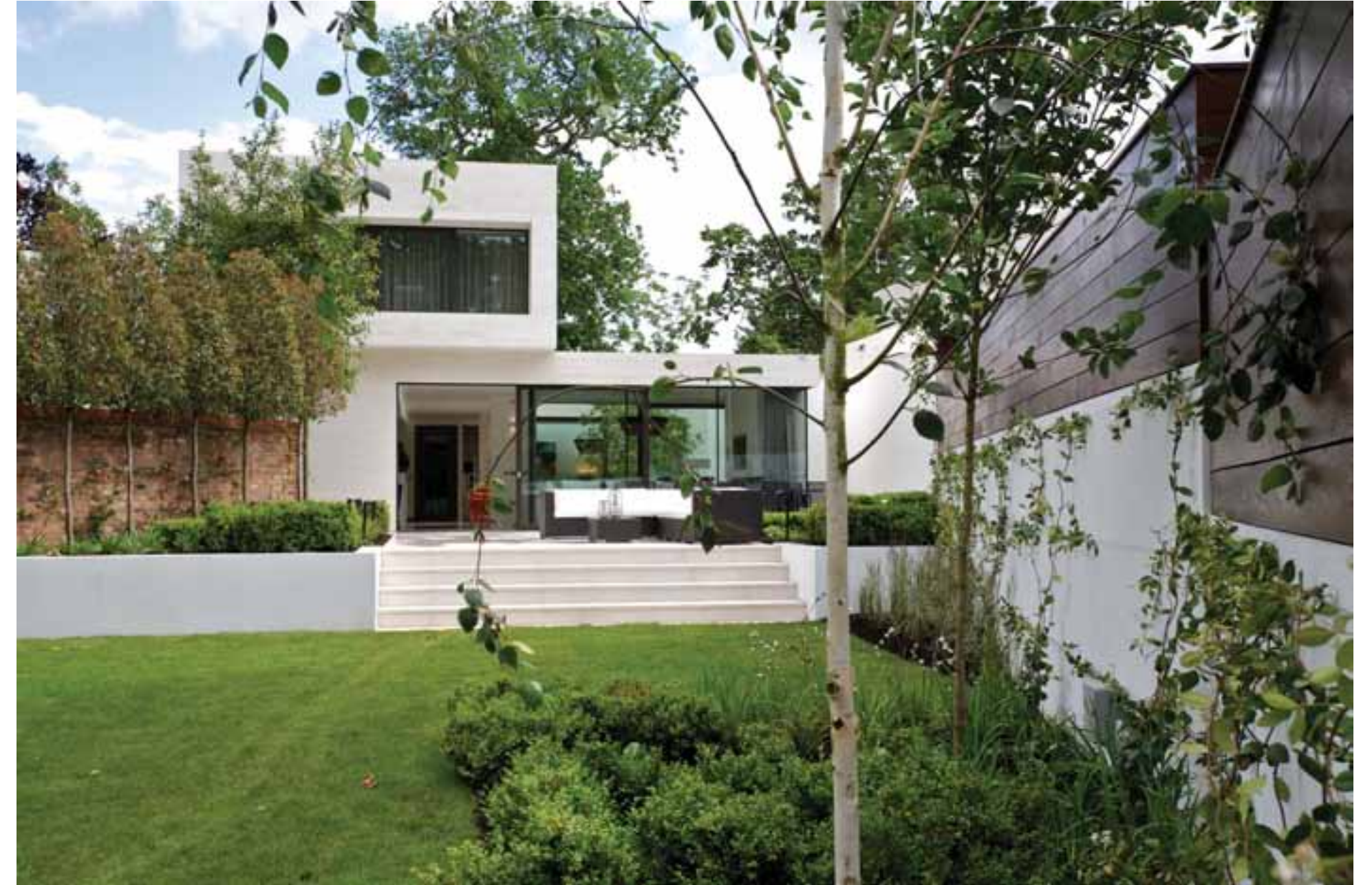
VIEW OF REAR TERRACE FROM GARDEN
